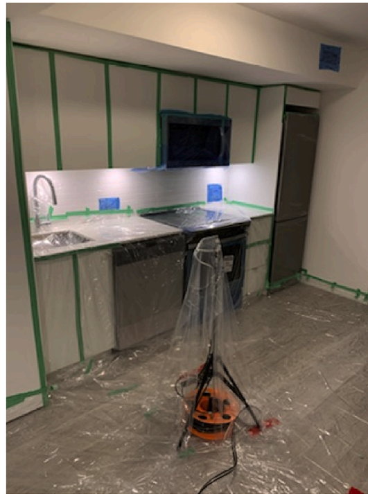
Fig. 1. Aerosolized sealant installation apparatus.
